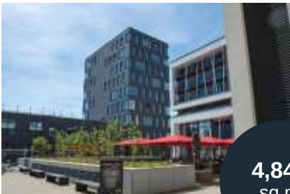
SOUTHLANE TOWER II ESCH-BELVAL
